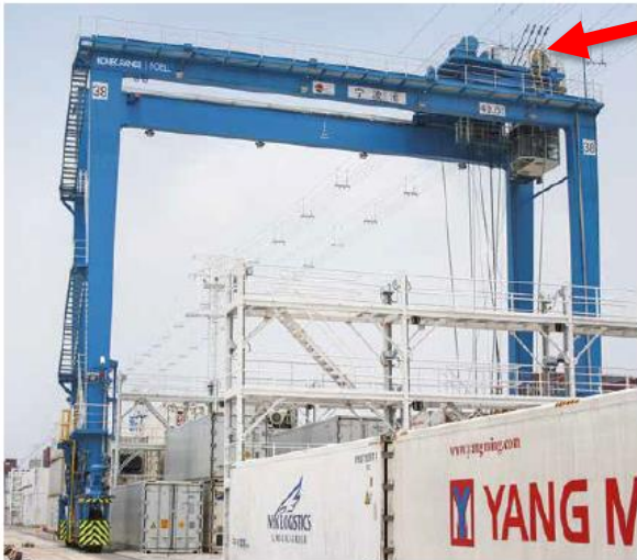
A Konecranes Noell RTG in action with an additional power option: overhead electrical trolley power.
